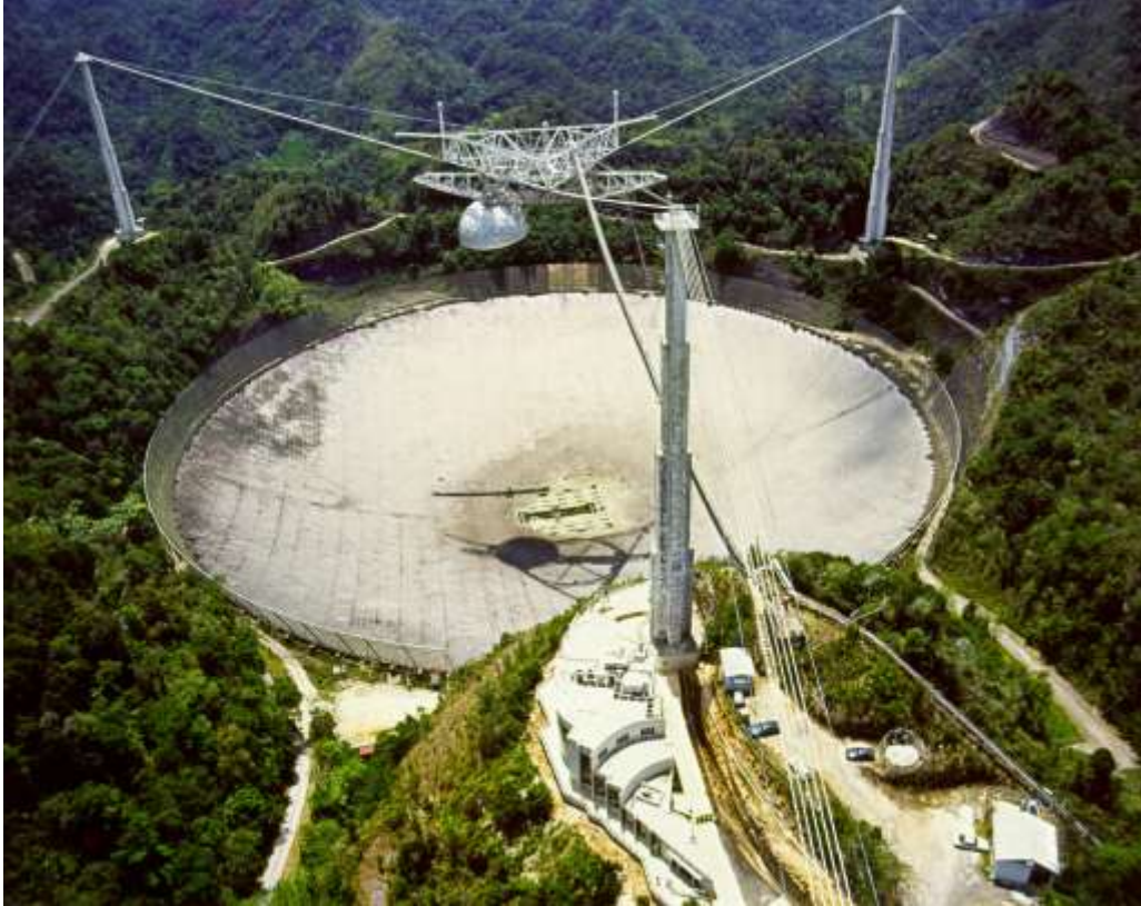
Figure 7. The Arecibo 1000-foot diameter radio telescope in Puerto Rico. Arecibo is the largest telescope on Earth. Schweiker, NOAO.
